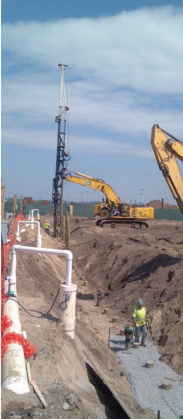
LEFT: C.A.C. Industries installed new sewers and the piles to support new infrastructure for Gateway Estates.
