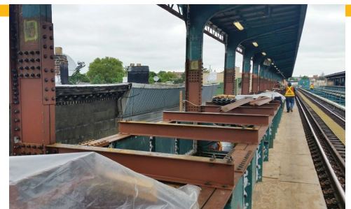
Pictured from left to right: The new 86th Street Station for the Second Avenue Subway (Schiaivone Construction and Skanska USA Civil / LK Comstock JV), Signal and track work at 75th Avenue Station on the E, F Queens Blvd Line (Railroad Construction), and Rehabilitation of the 4 Stations along the J, Z Lines in Brooklyn (E.E. Cruz & Co).
